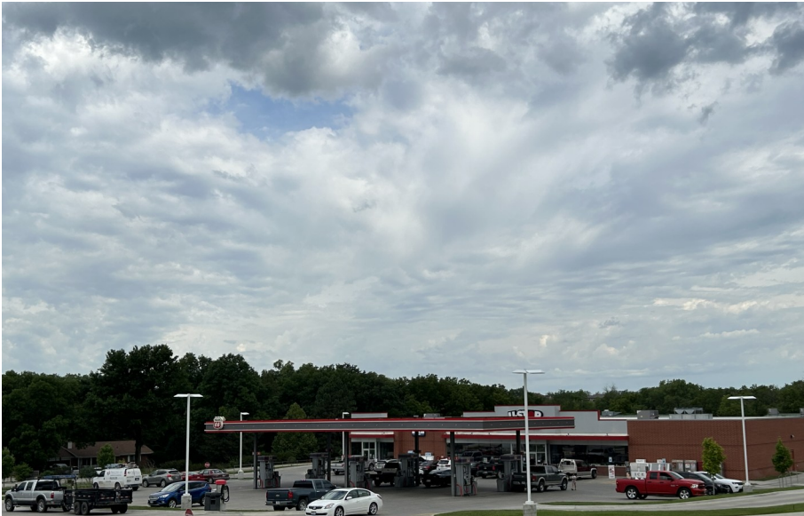
Photo 5.1: U-Stop Convenience, Hickman Source: Marvin Planning Consultants
